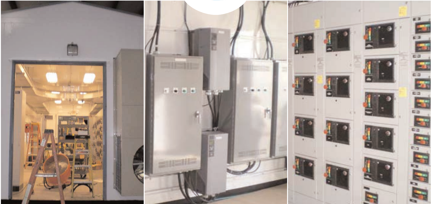
CUSTOM METAL BUILDING
